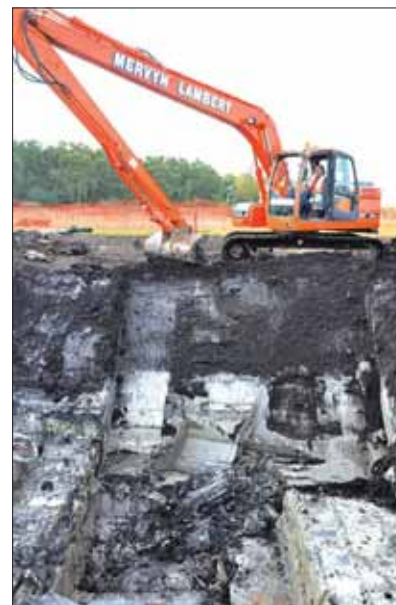
Plate 12: Long arm 360 machine used during the excavation
